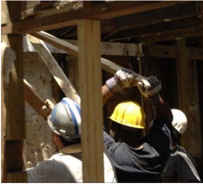
Training a crew to carefully salvage materials
