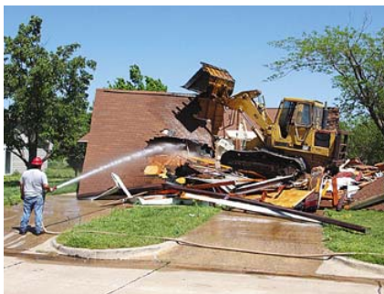
Deconstruction the old, unsustainable way
